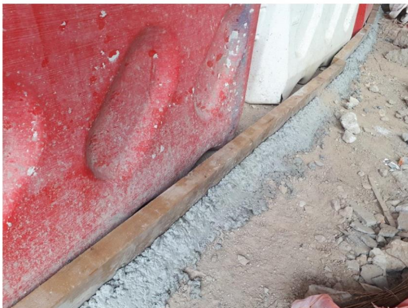
Figure A2: Earth bunded along the water barriers at P6 site area.
